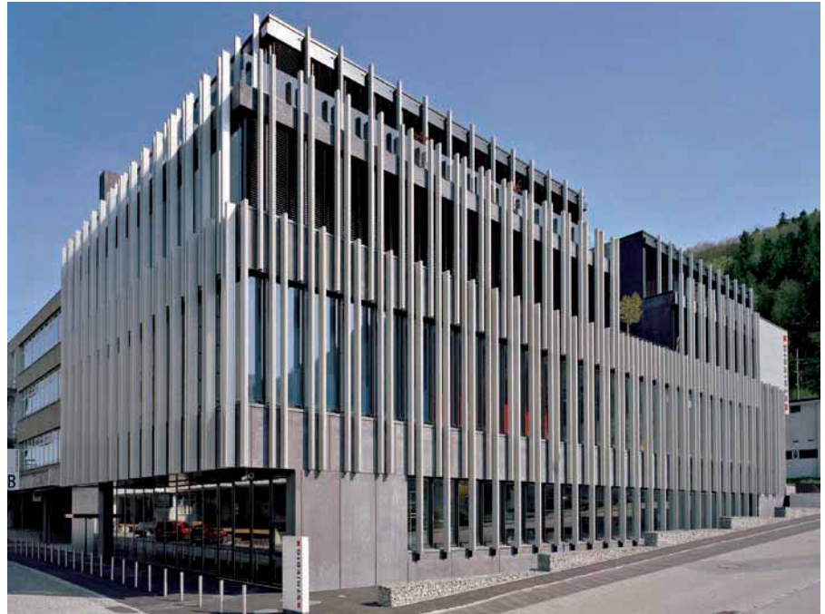
Built corporate identity: Vertical aluminium pilaster strips subdivide the front of our principal office in Littau in the near of Luzern, and establish a good reference to our products and market partners.
